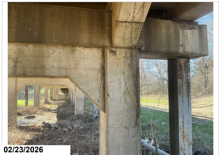
Bent # 10, column # 2 aheadface at the cap juncture has a shallow 4" spall with exposed reinforcing steel.
