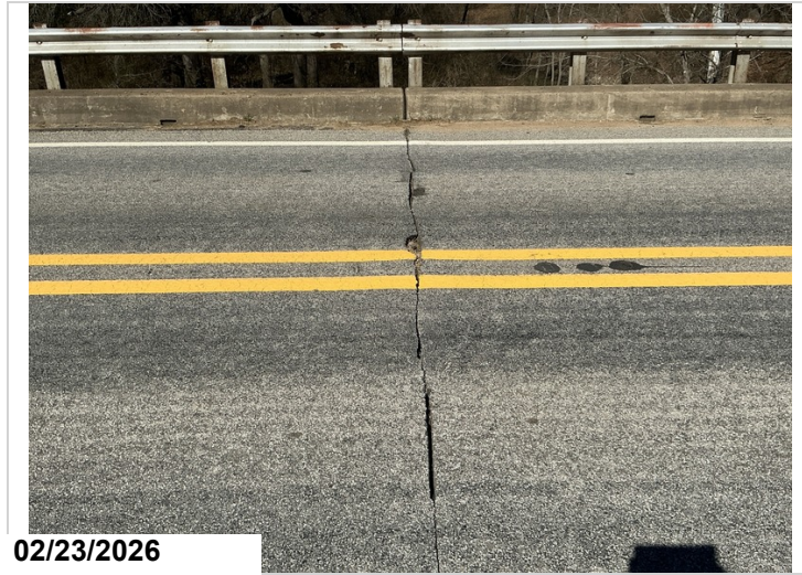
Bent # 4: 12" pothole over the bent in the westbound lane. 1SF CS3 spall
