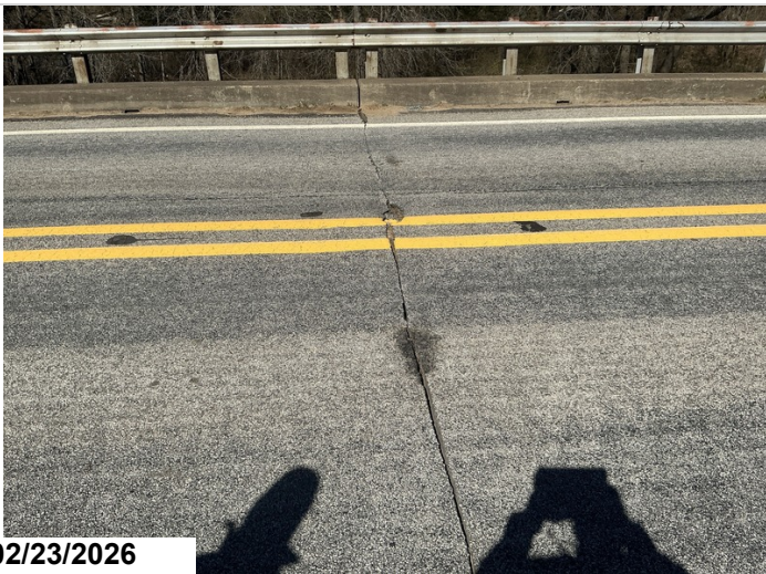
Bent # 2: 12" pothole over the bent in the westbound lane. 1SF CS3 spall
