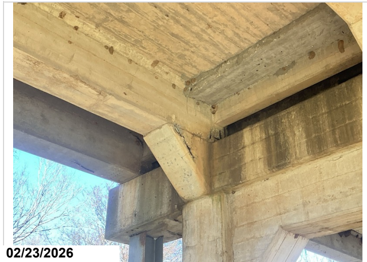
Span # 7, girder # 2 spalling with exposed reinforcing steel over bent # 8.
