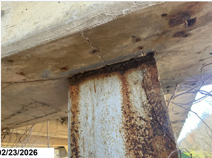
Bent # 11 left pile ahead flange has active corrosion with up to knife edge section loss at the cap juncture.
