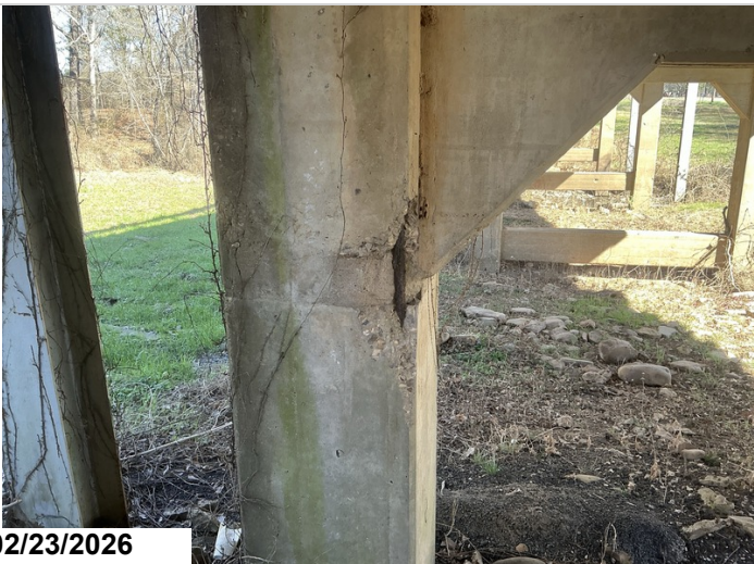
Bent # 2, column # 2 backface has a 24" high spall with exposed primary reinforcing steel. Exposed reinforcing steel has an estimated 1/16" section loss.
