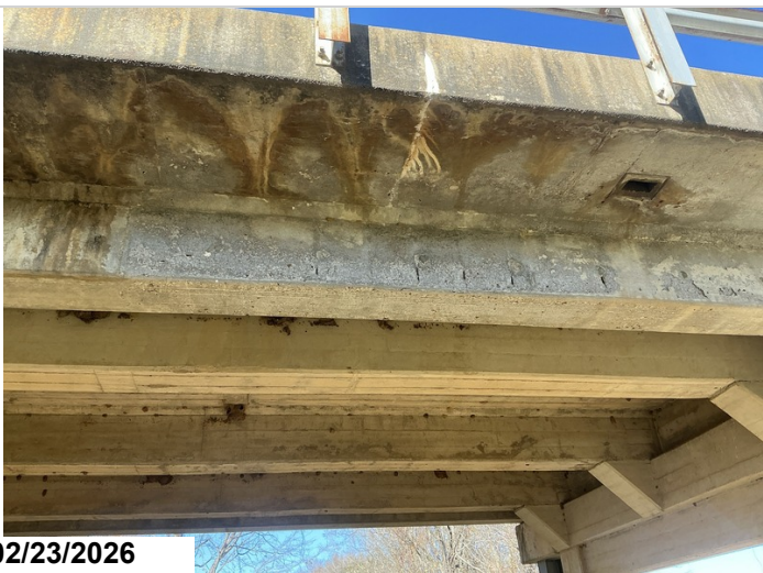
Span # 8, girder # 5 has scaling with several small shallow spalls with exposed reinforcing steel in the exterior face of girder.
