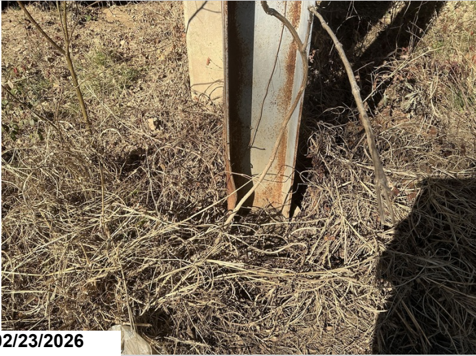
Bent # 7 right pile back flange has 1-1/8" out of plane bending to base of pile in an area approximately 16" high at the base of the pile.
