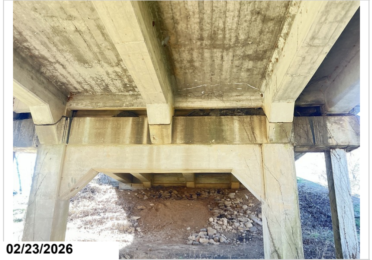
Bent # 2 asphalt on the bent cap.
