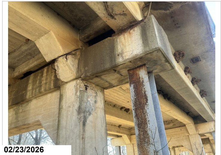
Bent # 8: the cap ahead face has a spall under girder # 1 that extends to the edge of the masonry plate. No loss of bearing area at this inspection. The cap haunch under girders # 2 & 4 have spalling that has been grouted in the past. Repairs have failed and are no longer in place exposing the reinforcing steel with up to initial section loss. The cap undersurface on both sides has several narrow width long shallow spalls with exposed reinforcing steel.
