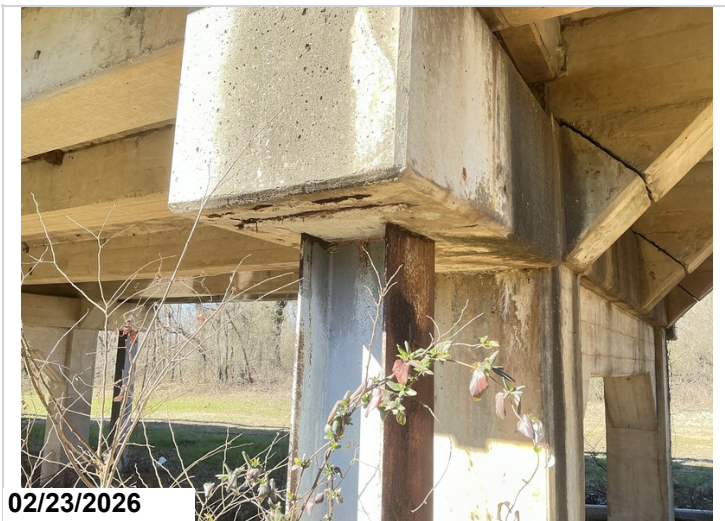
Bent # 10 right pile has a rust coating on the majority of the steel pile with up to 1/4" section loss at the cap juncture.
