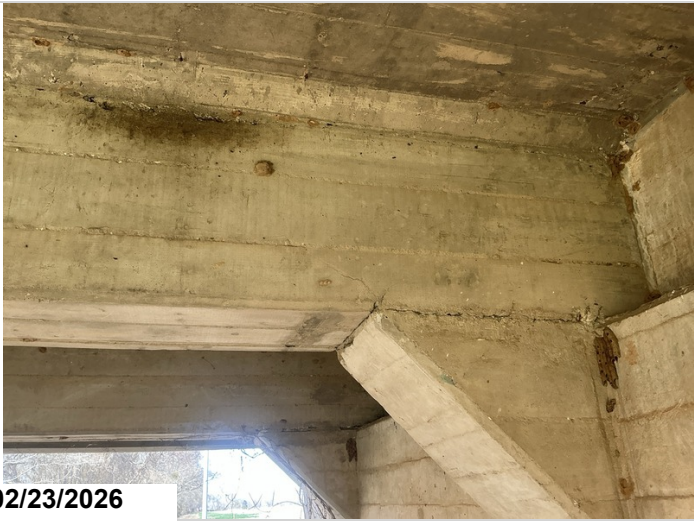
Span # 10, girder # 3 at bent # 11 has a diagonal hairline shear type crack.
