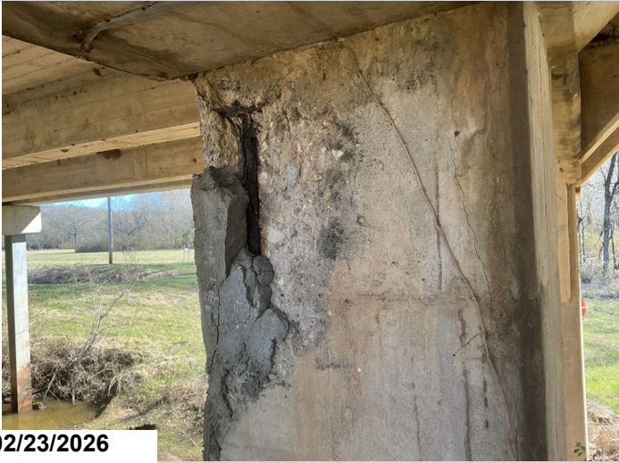
Bent # 8, column # 2 exterior face at the cap juncture has a 20" high x 12" wide spall with exposed reinforcing steel. Past repair to the spalled area has failed.
