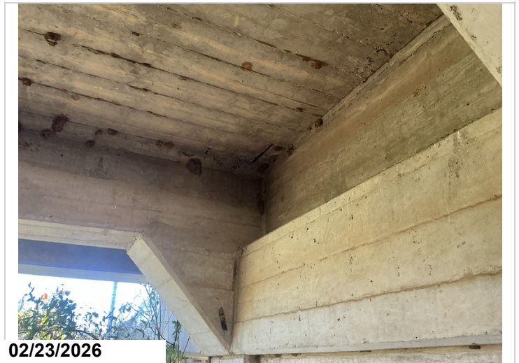
Span # 11 undersurface in Bay # 3 has shallow 10" long spall adjacent to bent # 11 with exposed reinforcing steel.
