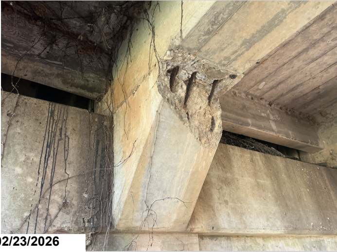
Bent # 2: the back face has a 14" spall with exposed reinforcing steel in haunch under girder # 2.
