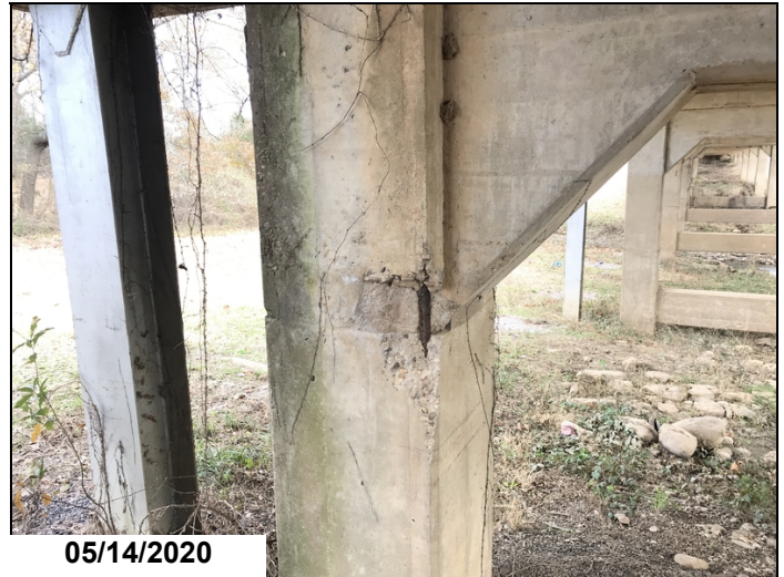
Bent # 2, column # 2 backface- Spalling with exposed reinforcing steel.
