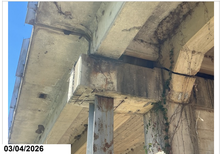
Span # 6, bearing # 5, bent # 6: bearing has heavy corrosion with layers of flaking rust/ section loss. The bearing has approximately 1" bearing area loss in a 5" long area due to spall in bent cap.
