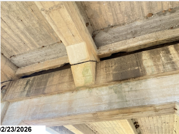
Bent # 8: spalling in the end diaphragm of bay # 2 & 3.
