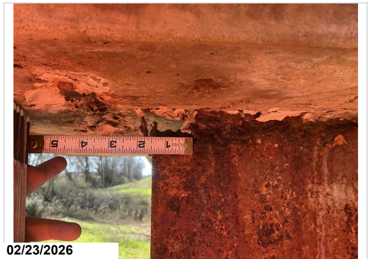
Bent # 8 right pile has active corrosion with a 1-1/2" long x 5/8" high hole rusted through the flange at the cap juncture. The left pile has 1/4" section loss at the cap juncture on the ahead face.
