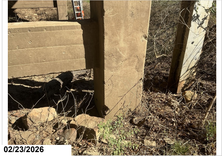
Bent # 4, column # 2: there is honeycombing/ concrete deterioration at the base of column.
