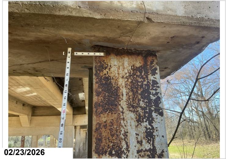
Bent # 10 left pile has active corrosion with knife edge section to the ahead flange with a 1/2" hole and a 1" hole rusted through the flange at the cap juncture.
