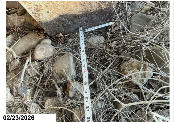
Bent # 11, left : Base of pile at ground level has heavy corrosion with thick layers of flaking rust to web and flanges in an area approximately 12" high. Flanges have knife edge section loss along tBent # 11, left : Base of pile at ground level has heavy corrosion with thick layers of flaking rust to web and flanges in an area approximately 12" high. Flanges have knife edge section loss along the edges. The ahead flange in the affected area is reduced to 5/16" thickness and has a 1/2" hole rusted through.
