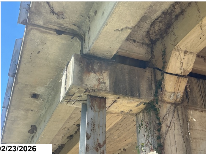
Span # 6, bearing # 5, bent # 6: bearing has heavy corrosion with layers of flaking rust/ section loss. The bearing has approximately 1" bearing area loss in a 5" long area due to spall in bent cap.
