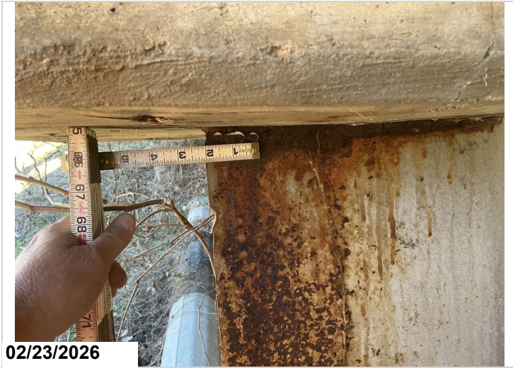
Bent # 11, left: The back flange has a 2" x 1/2" hole rusted through at the cap juncture.
