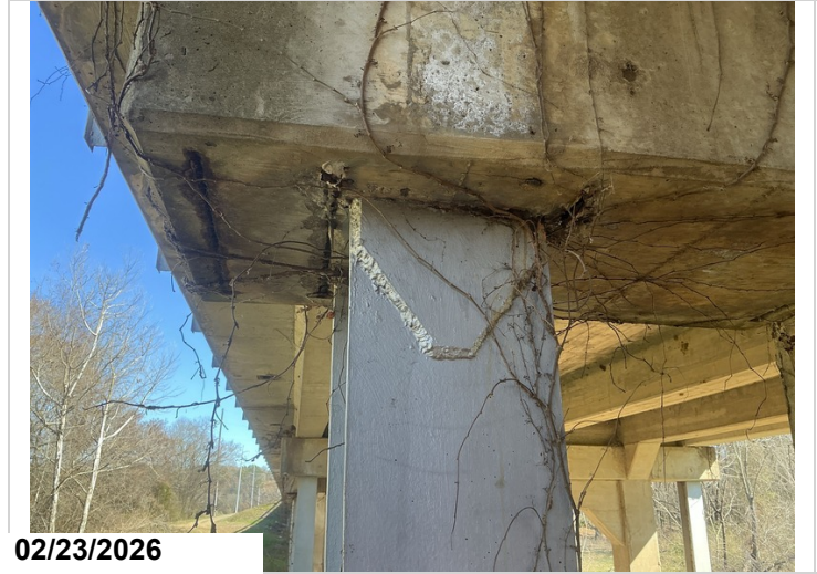
Bent # 2, left: The undersurface of cap on left end has two 18" long shallow spalls with exposed reinforcing steel.
