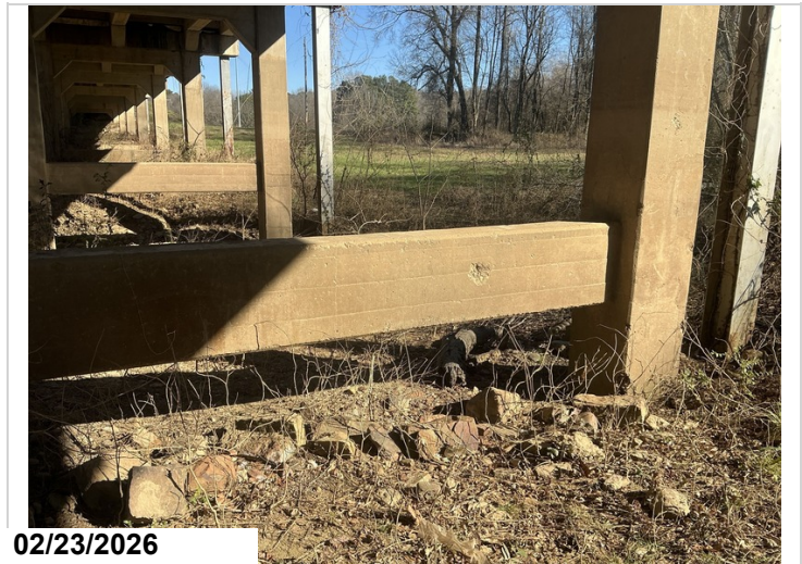
Bent # 4 strut backface has a 6" shallow spall with no exposed reinforcing steel
