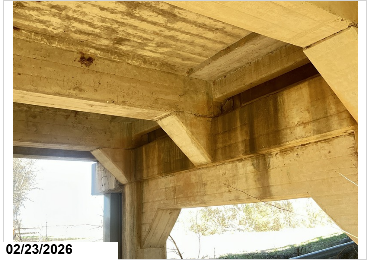
Span # 9, girder # 3: 14" long spalling with exposed reinforcing steel over bent # 10.
