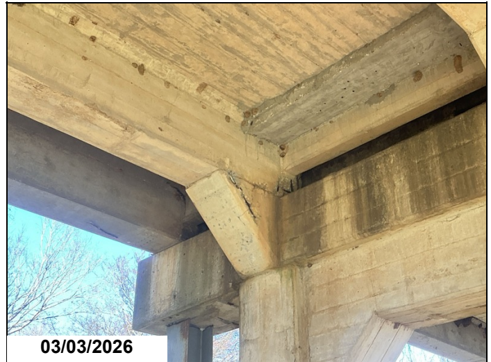
Span # 7, girder # 2 spalling with exposed reinforcing steel over bent # 8.
