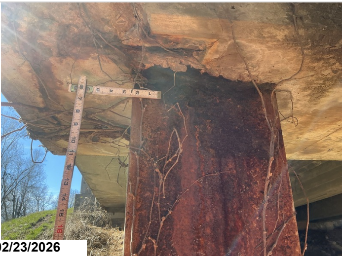
Bent # 2 right pile has active corrosion up to knife edge section loss at the cap juncture with an area of complete section loss to ahead flange that is 2-1/4" long x 1/2" wide.
