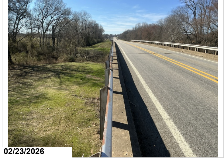
Span # 9, right: the bridge railing has minor collision damage in an area approximately 12' long that has caused out of plane bending to the railing and bent one post out of plumb.
